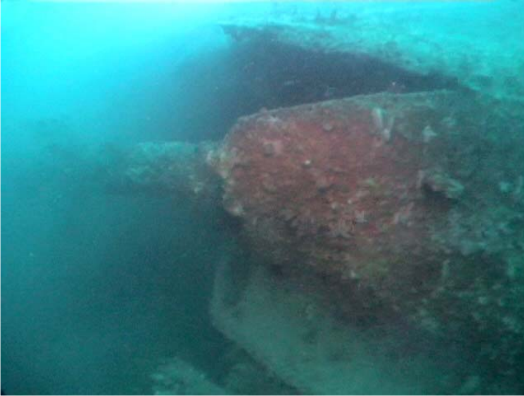
X4/3 - Torp hole to left, shaft center left. Forward edge of hole just below shaft exit point.
