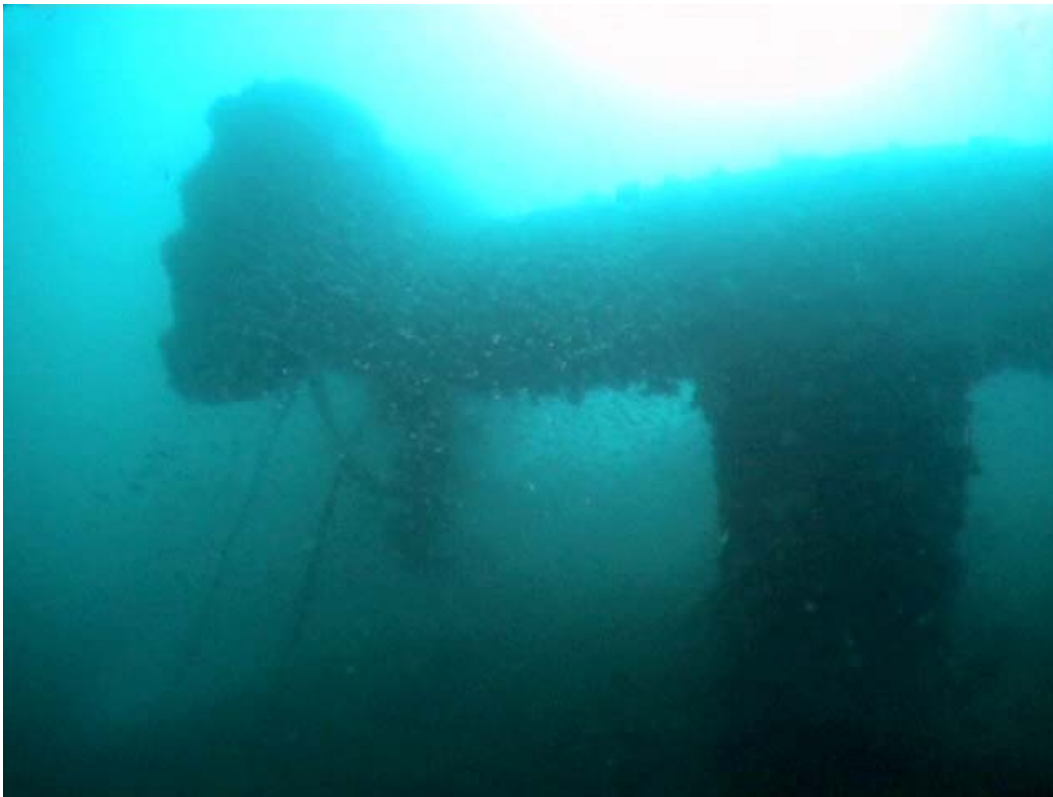
Chipped blade on inner Port propeller; right, outer strut of its intact supporting A-Bracket.
