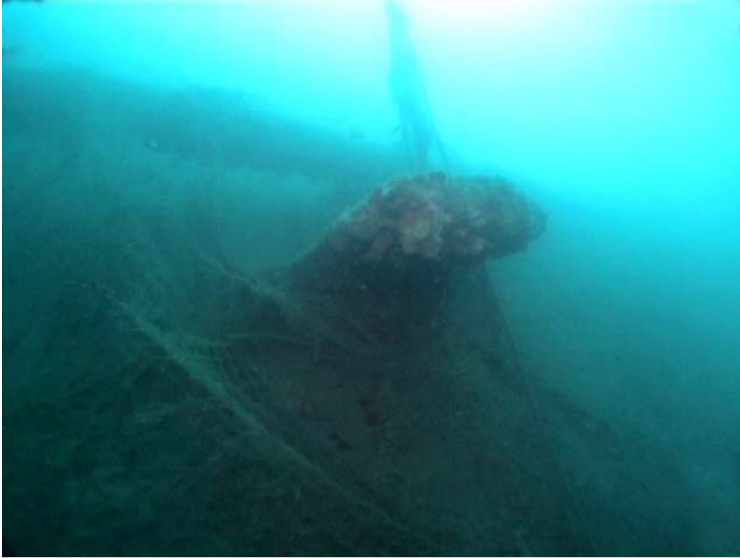
D1- Stub of inner strut of Port outer shaft A-Bracket. Inner Port propeller shaft upper left.
