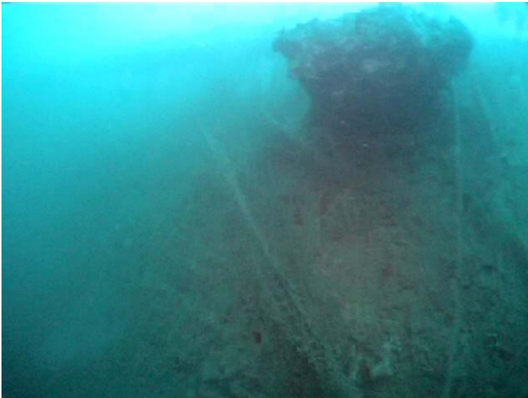
D2 - Only a short stub remains of the inner strut of the outer Port shaft A-Bracket.
