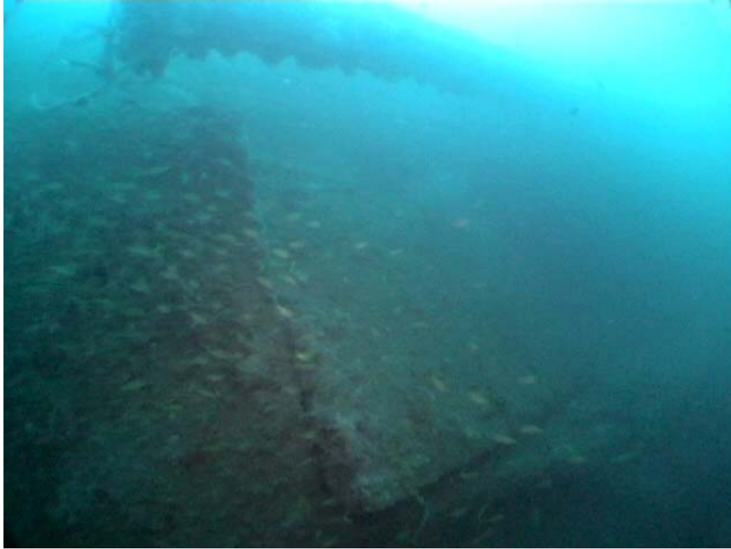
X4/7 - Aft edge of same collapsed hull plate as seen in X4/6 is just below flange on outer shaft end.
